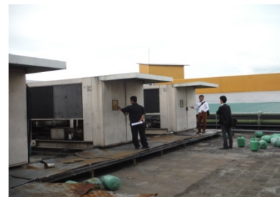
Field survey – building roof top
